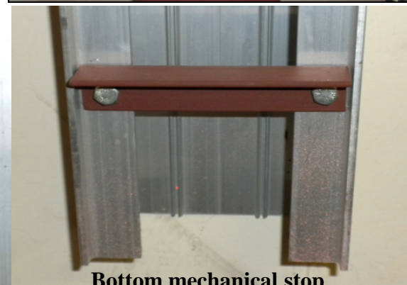
Bottom mechanical stop
